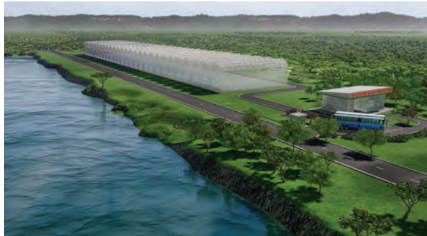
LEFT AND BELOW LEFT: Artist's impressions of Gallant Obayashi Green Agritech Park.
