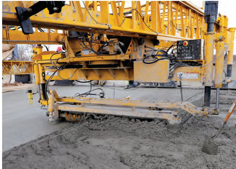
The new screed can pave up to 31.7 m in width and advance up to 1.2 m in a single pass.
