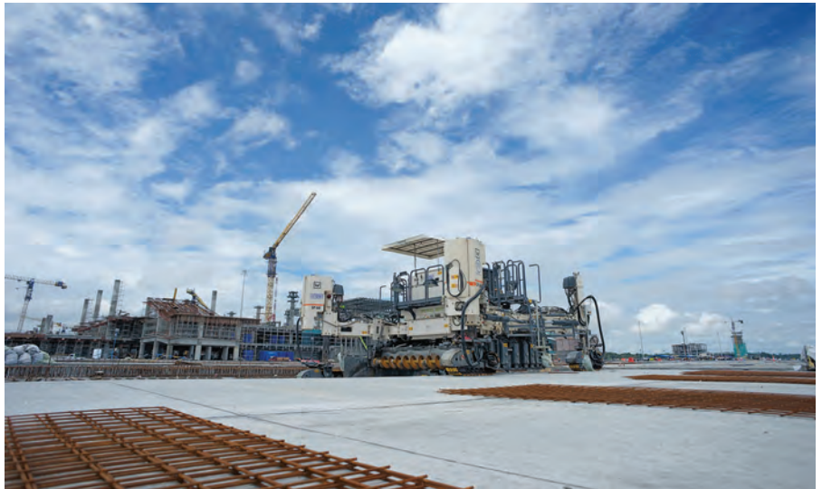
ABOVE AND BELOW: Wirtgen slipform machines on the new Yogyakarta International Airport project, paving the 3,250-m-long, 45-m-wide runway, its taxiways, and the apron.
