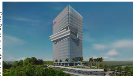
BELOW: SunTec's new campus at Technocity, Pallipuram in India, is one of the projects where Surbana Jurong had leveraged its BIM capabilities.
