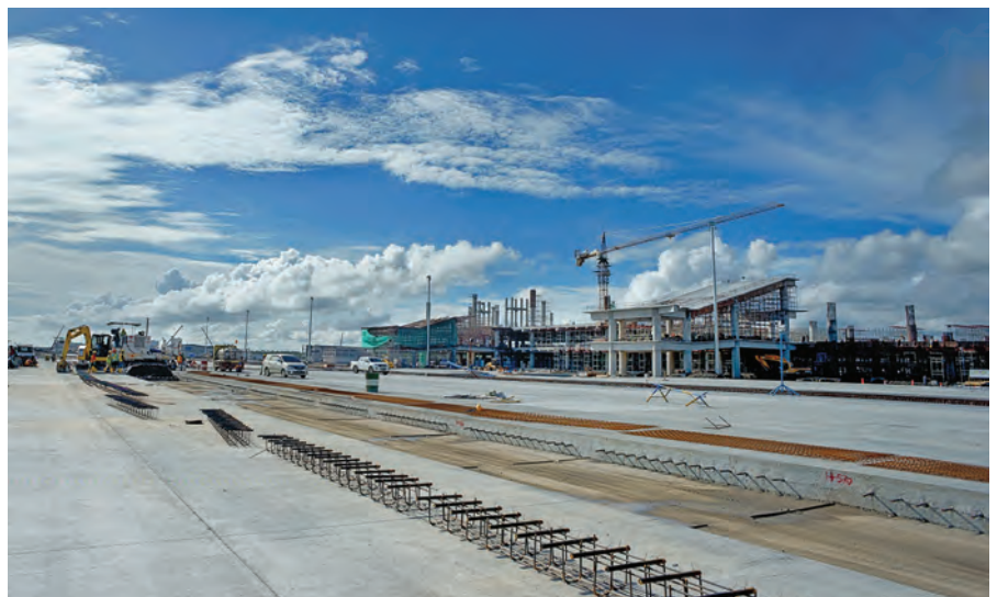
ABOVE AND BELOW: Wirtgen slipform machines on the new Yogyakarta International Airport project, paving the 3,250-m-long, 45-m-wide runway, its taxiways, and the apron.
