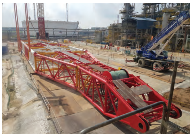
The boom booster kit on the job site.
