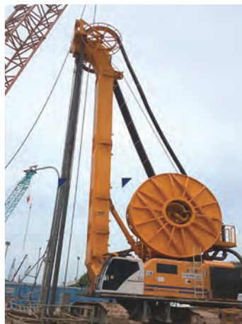
SC40+HDS80 in C886 Tunnel at Marina Bay Project in SINGAPORE
