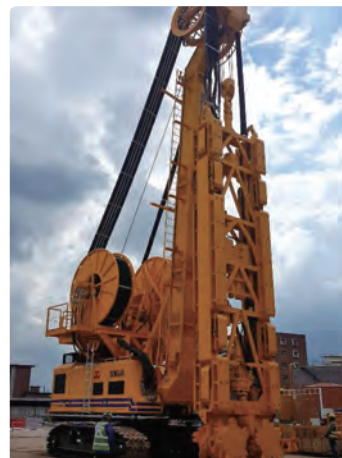
SC40+HDS80 in UGS Construction Project in SINGAPORE
