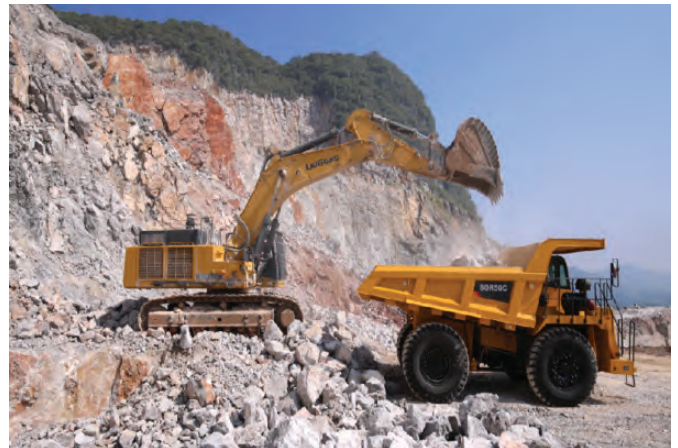
BELOW: LiuGong machines working at a quarry.
