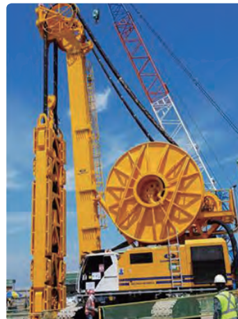
SC40+HDS80 in Contract T7 Project in SINGAPORE
