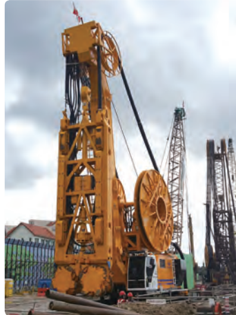
CSC40+HDS80 in T312 Sungei Bedok Station Project in SINGAPORE
