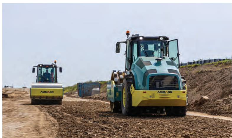
TOP AND ABOVE: Vinci Construction Terrassement is currently working on a new section along the high-speed rail line between the Stuttgart airport and Wendlingen. The construction required earthworks for a 5.4-km ICE track and 7.5 km of side roads.
