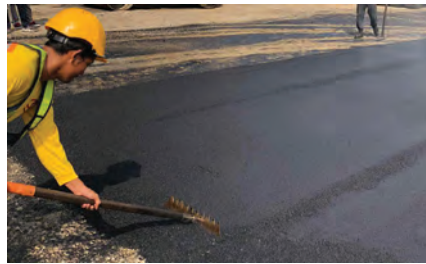
ABOVE AND LEFT: A pilot test for the recycled plastic road was conducted at the end of last year on a 1,500-sq-m area in General Trias, Cavite.
