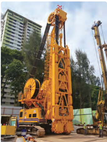
SC40+HDS80 in Contract C883-CCL6 Project in SINGAPORE
