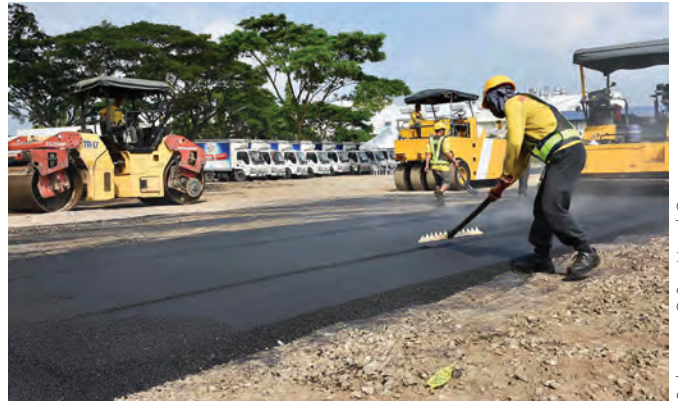
ABOVE AND LEFT: A pilot test for the recycled plastic road was conducted at the end of last year on a 1,500-sq-m area in General Trias, Cavite.
