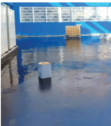
ABOVE AND LEFT: The floors in the corridors and on the stage were waterproofed with Mapei Plastimul PU membrane.
