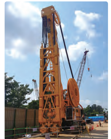
SC40+HDS80 in Contract T10 Project in SINGAPORE
