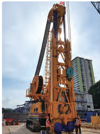
SC40+HDS80 in Contract C883-CCL6 Project in SINGAPORE
