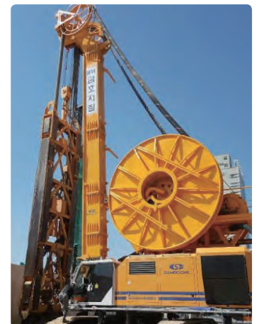
SC40+HDS80 in Gwang Ann Construction Project in SOUTH KOREA
