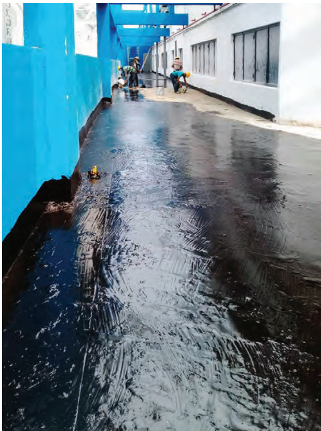
ABOVE AND LEFT: The floors in the corridors and on the stage were waterproofed with Mapei Plastimul PU membrane.
